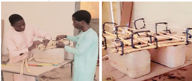
Figure 2: Preparation of bamboo reinforcement
